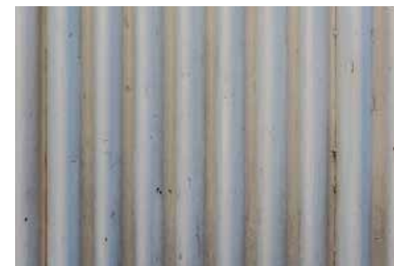
Corrugated metal roofs for sign kiosks
