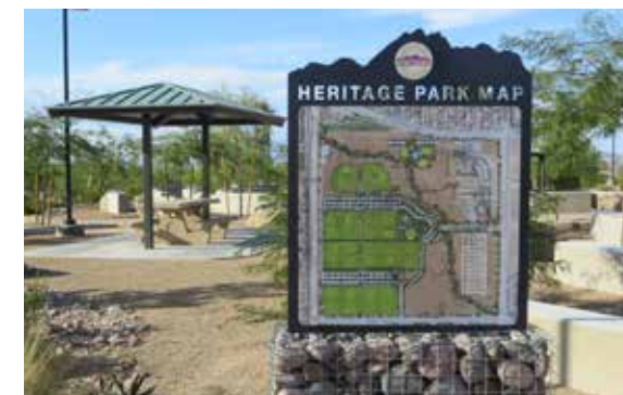
Use of gabion wall at sign base with cutout top
